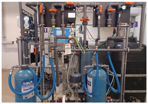
In 2024 the Department of Geoscience had a new water system installed, ensuring highquality TYPE 1 water according to the ASTM standard <u>D1193-99e1</u>. The system is remarkable because it uses a minimum of resources (energy, salt and water) compared to older technologies. In total 600 liters can be produced per hour. Some of the already processed water is recirculated, providing a stable and very clean demineralized and ion-free water supply for our laboratories.
